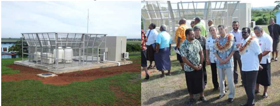
Wind profiler (weather observing equipment) (Provided by JICA) Facility tour (Provided by Embassy of Japan in Fiji)
